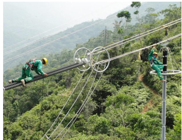
Figure 15 : Installation of 420kV NGLA in Columbia
