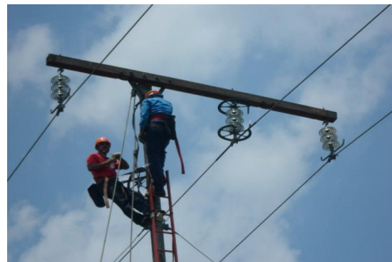
Figure 12. Installation of SAS by Malaysian DSO
