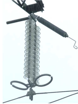
Figure 11. 225kV EGLA design for live line installation. Courtesy of RTE.
