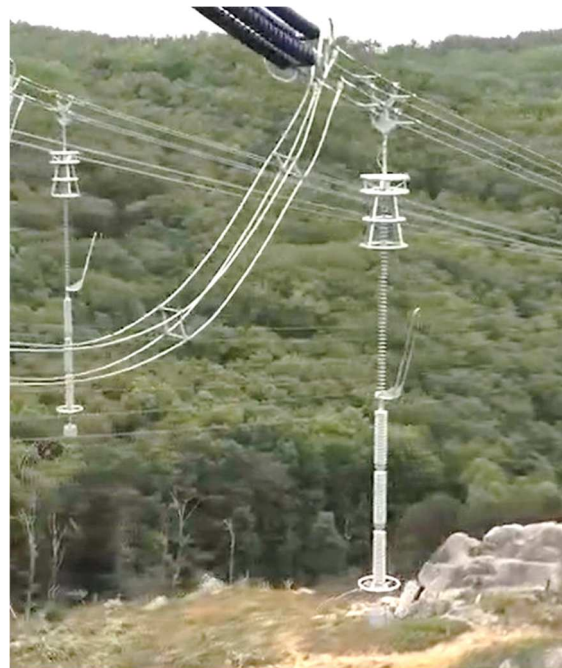
Figure 15. 765kV EGLA "rigid gap" hanging from the conductor of a dead-end insulator
