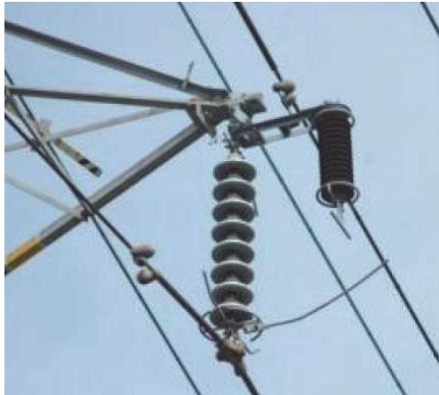
Figure 5. Conventional EGLA type (1st generation) (2)
