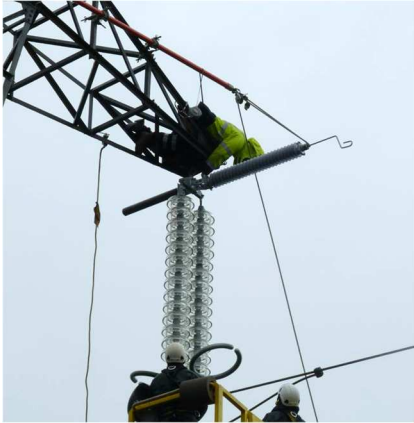
Figure 10. 225kV EGLA design for live line installation. Courtesy of RTE.
